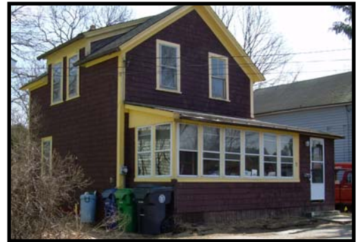
One of our clients home prior to demolition
